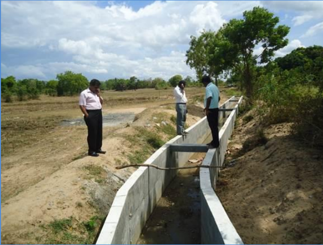
Improvements to Adachakal Tank Channel System
