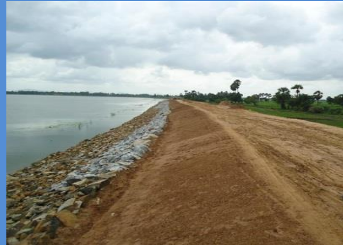
Rehabilitation of Damage Bund at Kadukkamunai Kulam
