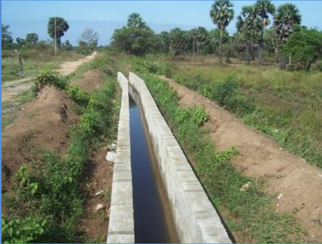
Improvements to Head Works and Channel System of Andan Kulam
