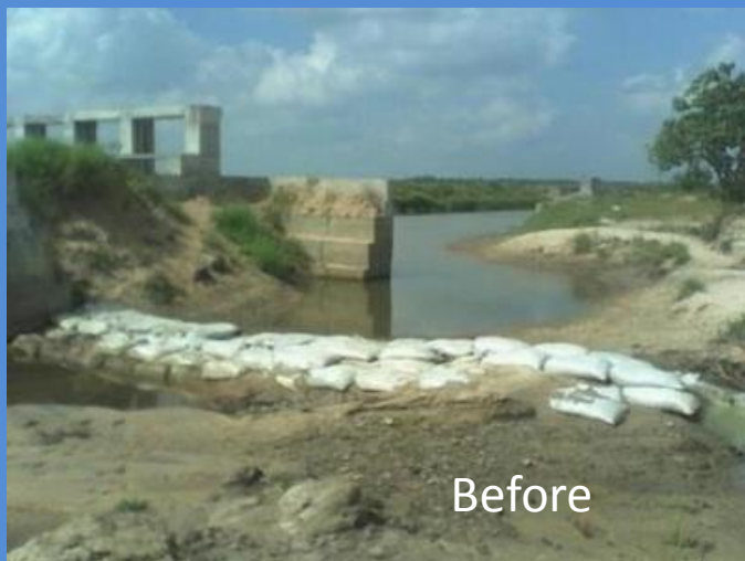
Construction of concrete Lining channel and Retaining wall in Chadayanthalawa Scheme
