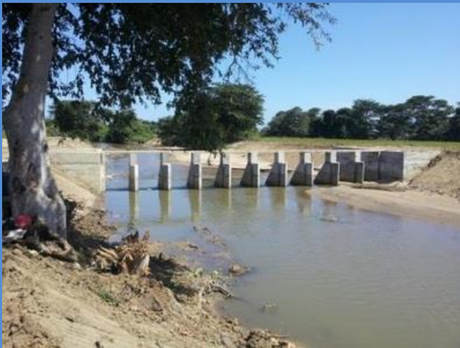
Improvements to Pavankai Anicut and Access Road
