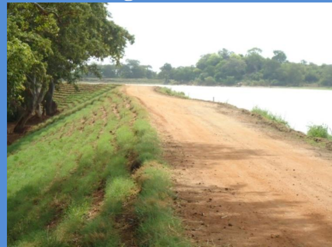
Improvements to Head Works and Channel System of Periya kulam
