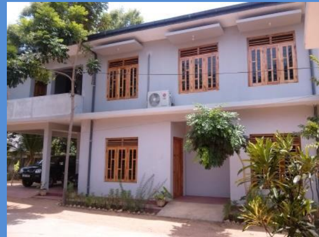
Rehabilitation of Soil Lab at DDI's office Kalmunai
