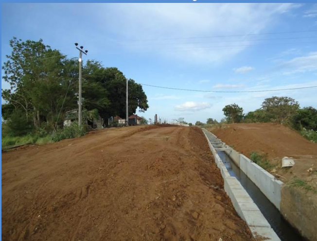
Improvements to RB main channel at Mathurankerni Kulam
