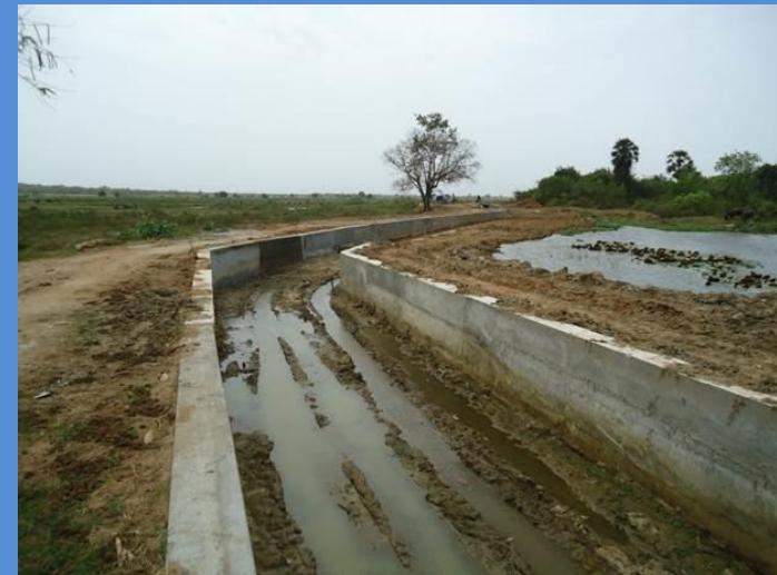
Improvements to Tharavai Kulam main Channel
