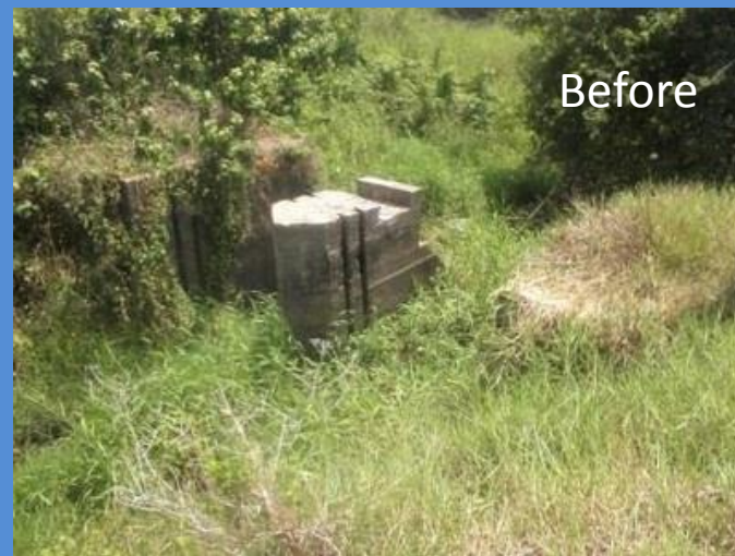
Construction of Regulator and Retaining wall in Sagamam Scheme
